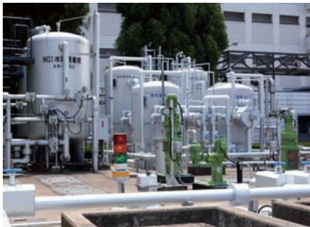
System for treating wastewater from research for reuse at the Central Research Laboratories
