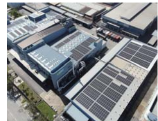
Solar panels installed in Malaysia
