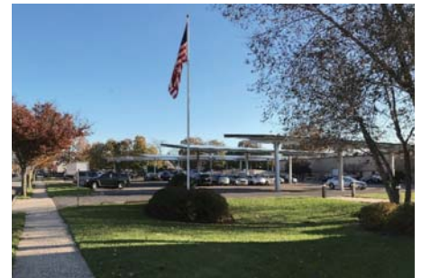
Solar panels installed on the roof of the Carlstadt R&D site's parking structure
