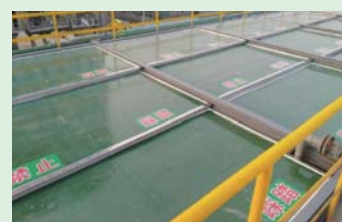
Graywater pit after sealing and treatment to remove odors
