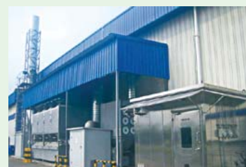
New system for thermally decomposing and deodorizing VOCs
