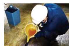
Sealing leaks
