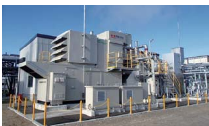
Natural gas turbine-powered cogeneration system at the Kashima Plant
