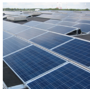
Solar panels in Wavre, Belgium
